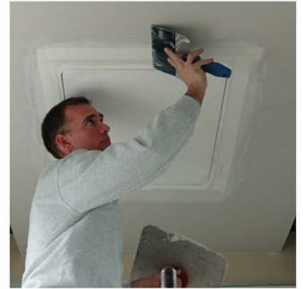
3. Smooth drywall tape and compound with a taping knife.
