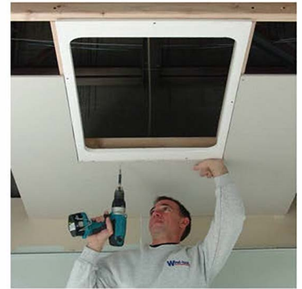
3. Hang drywall around the panel frame.
