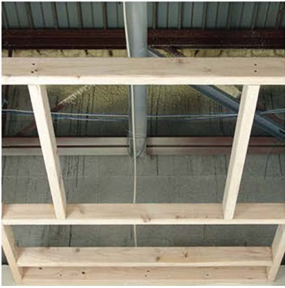
1. Frame out location of the panel.
