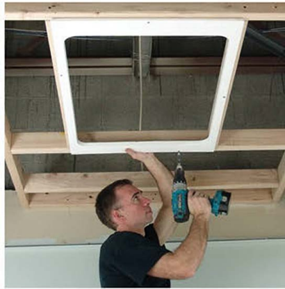
2. Affix panel frame by screwing it into ceiling frame using pre-marked divots.
