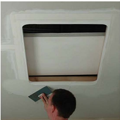
4. Apply second layer of mud and smooth with a taping knife.
